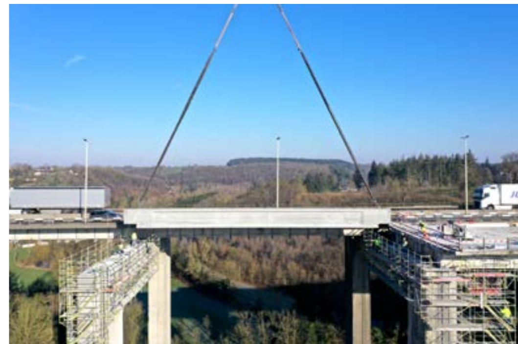
Viaduc Huccorgne (E42/A15) ©SOFICO-DETIFFE
