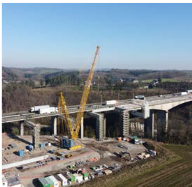
Viaduc Huccorgne (E42/A15) ©SOFICO-DETIFFE
